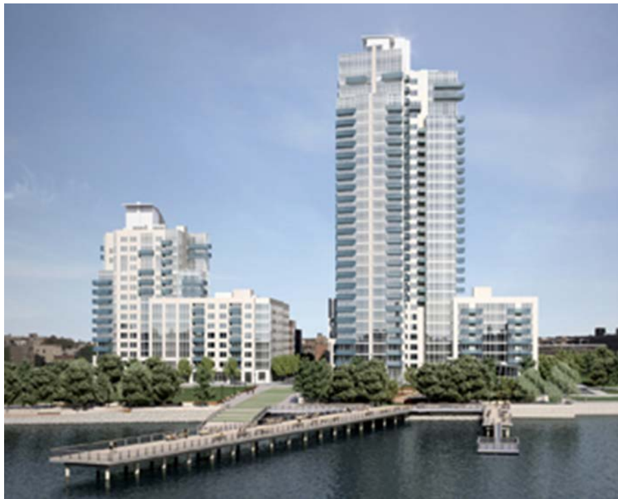
Edge Condominium (location of 9 units)
